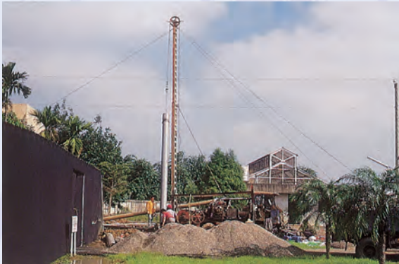
▲ 鑿井工程 Well drilling engineering
